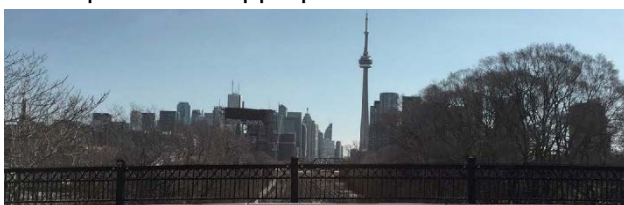
Above: Before installation of bridge barrier (Stachan Ave Bridge looking eastward)
