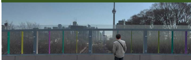
Above: After installation of bridge barrier (Stachan Ave Bridge looking eastward)
