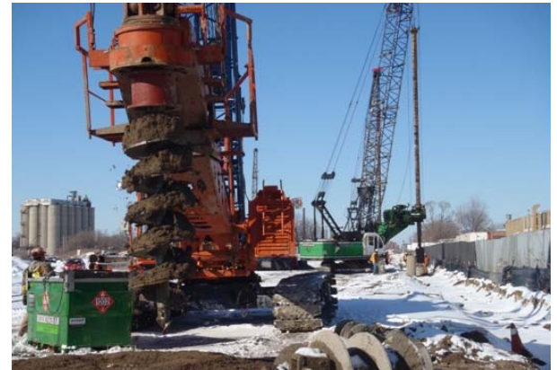
Crane-mounted augers (drills) remove soil from pipe piles
