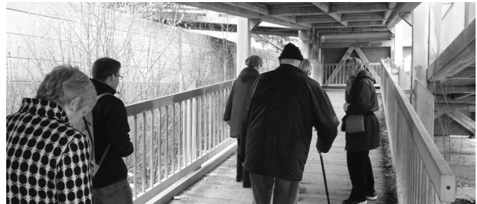
Four members of the York West Active Living Centre provide comments on a local pedestrian bridge.
