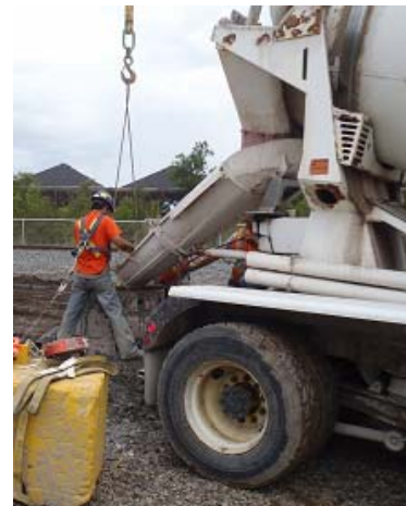
Construction worker pouring concrete in steel caisson.
