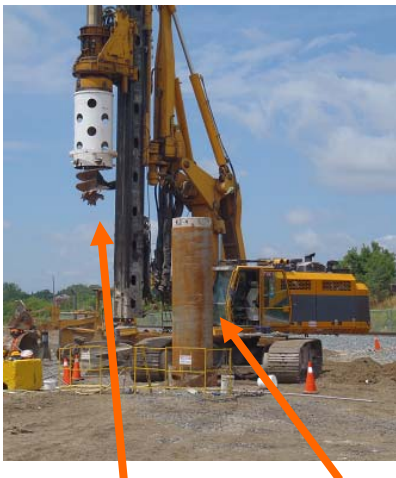
Drill rig with drill bit attached. Steel caisson (liner).
