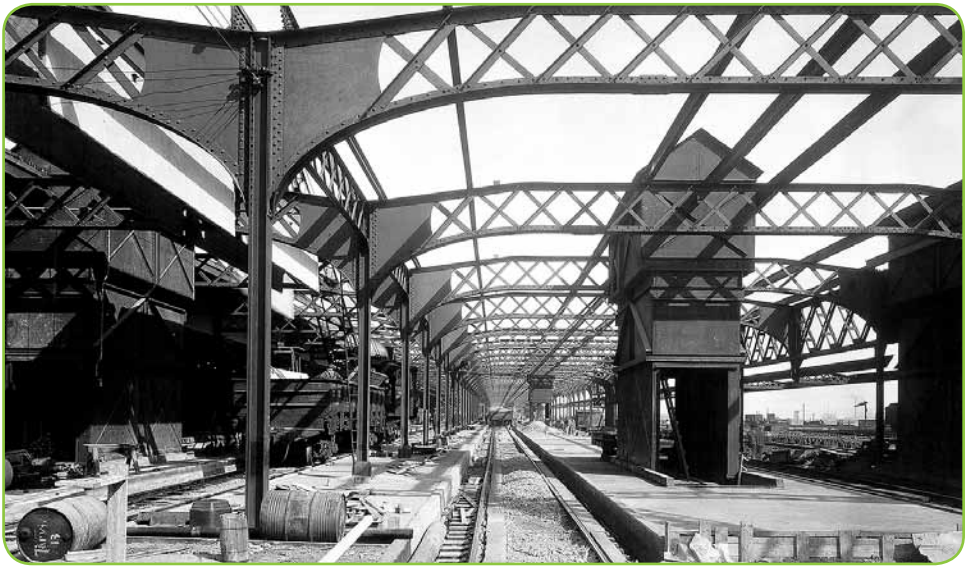
Early construction at Union Station.
