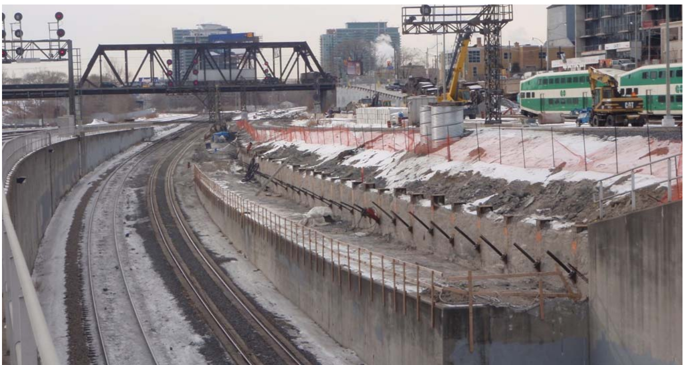
Retaining wall construction located east of the Spadina underpass (facing west).
